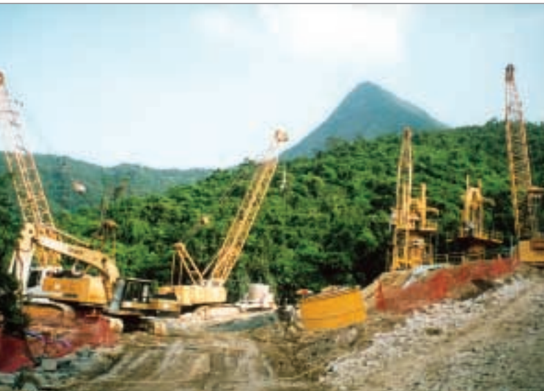
Construction of Road T7 in Ma On Shan (Bored Piling Works)
