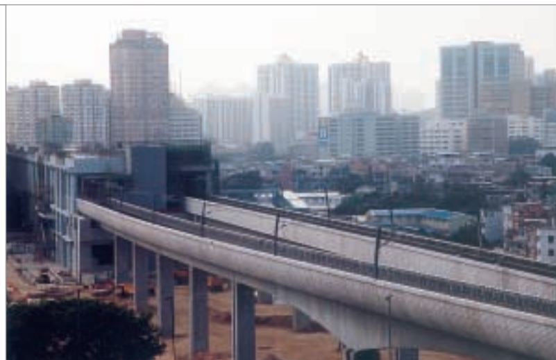
KCRC West Rail (Yuen Long Station)
